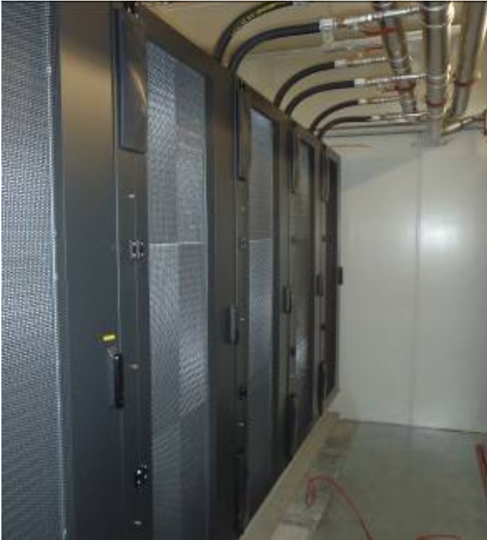
Up to 35 KW Per Rack Passive Coil
