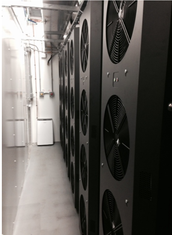
Up to 55 KW Per Rack w/Active Fan Kits
